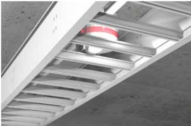
The sensor is completely obstructed by the obstacle
