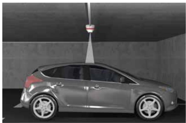
The sensor is properly mounted in the middle of the parking bay above the car
